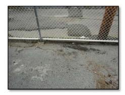
In order to control the invasion of the tree roots, a trench (one meter deep) was dug along the fence and Biobarrier was set in place making sure that it would extend up to the surface at ground level.
