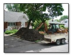
The pipe joint on the homeowner's property and the connection to the municipality's sewer pipe were then wrapped with Biobarrier and secured with tie wraps. The trench was refilled with the soil that had been removed.
