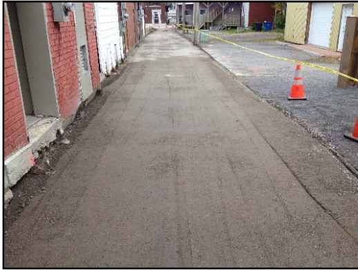
Compacting the crushed stone and stone dust.
