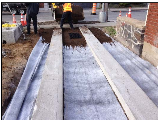
Positioning of a geo-textile covering the space around the concrete slabs.
