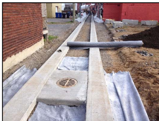
Positioning of a geo-textile covering the space around the concrete slabs.
