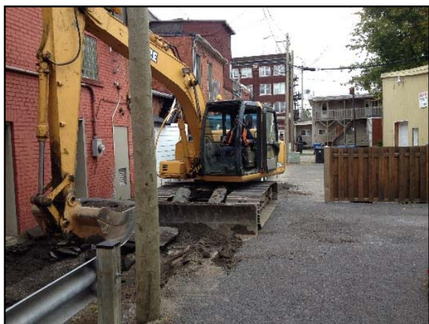
Removal of the asphalt surface.
