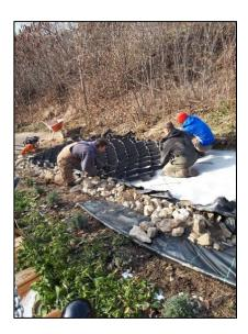
Geocells filled with sand/crushed stone and anchored with 21" J-Pins.
